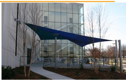
The tension membrane shade structure is a two sail overlapping structure that adds much needed shade to LabCorp's renovated outdoor dinning area. The sails enhance the overall aesthetics of the existing building while complementing the new updated addition. The three point sails are Commercial 95 shade cloth in Turquoise and Aquatic Blue to complement the LabCorp logo. This fabric is distributed by local manufacturer Glen Raven Mills.
