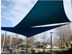
This structure is Wind Rated for 170 mph with cover off and 120 mph wind load with cover on.
