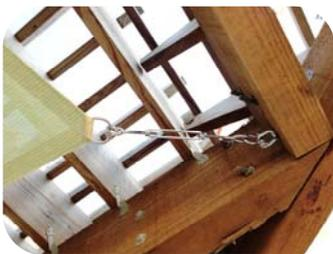
**Suggested Post Attachments:** Eyebolts, pad eyes (mounting brackets), eye screws, and turnbuckles are recommended depending on the post type.
